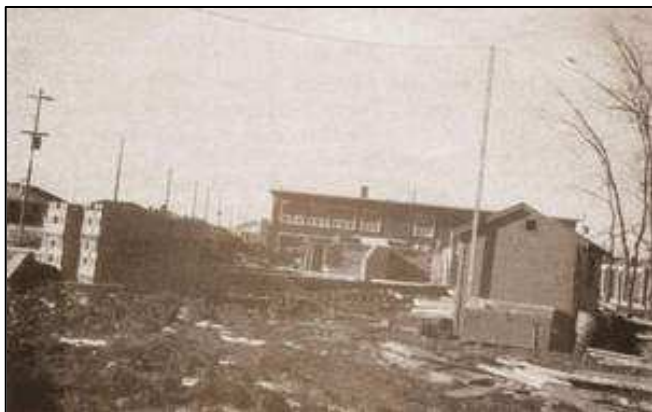
Resurrection Church under construction, Fall 1959
